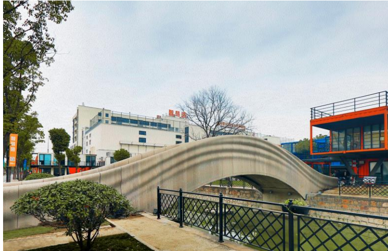
Figure 4. 3D printed bridge in Shanghai. Source: [60].
