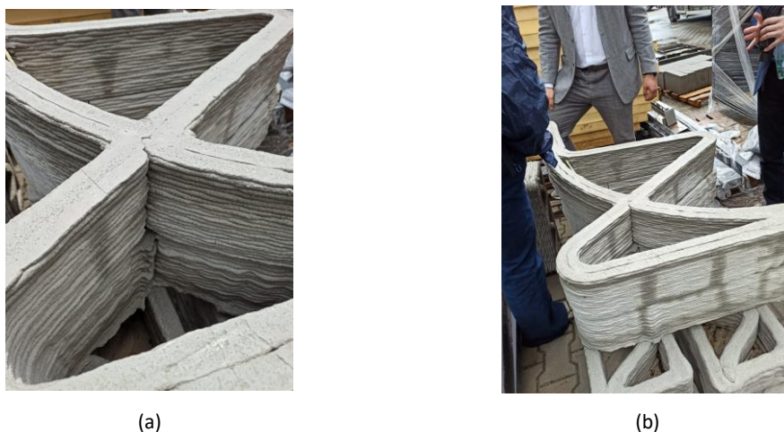
Figure 8. 3D printed elements developed in the framework of the project: (a) the element with visible layers, (b) the element compared to the human scale. Source: Own.
