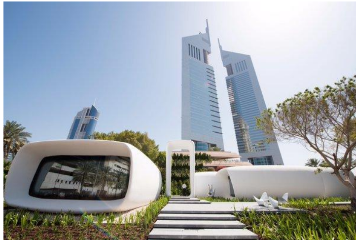
Figure 6. 3D printed office building in Dubai. Source: [70].
