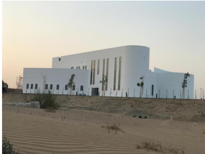
Figure 5. 3D printed administrative building for Dubai Municipality. Source: [64].
