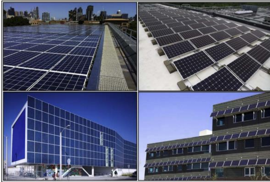
Fig. 3. Flat and tilted panel installation over building roofs and facades. Source: [10]
