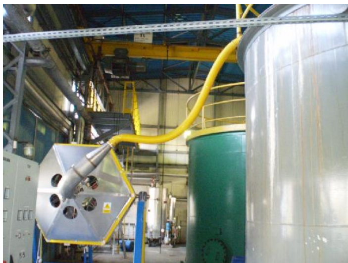
Fig. 6. Installing the activator on the real object Source: Author's
